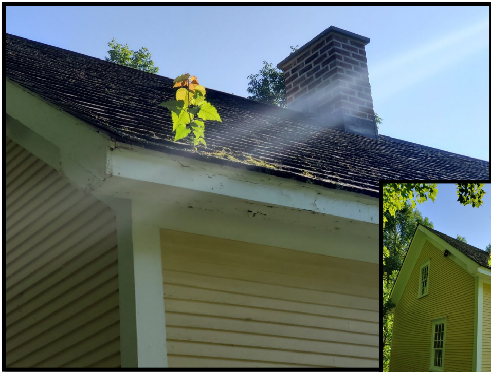
Removed deteriorated wood shingle roof that was leaking
